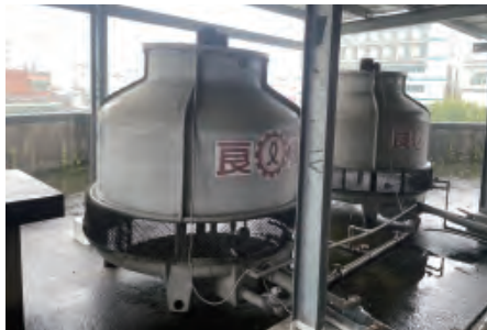
Counterflow cooling water tower
