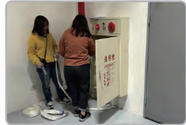
Fire hydrant operation
